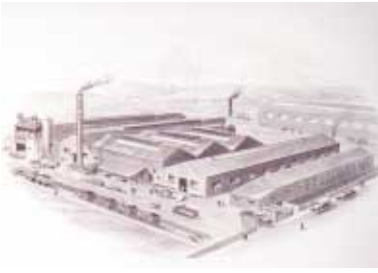
Climax Works 1930's
