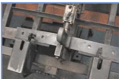
Welding preparation - Automatic flight assembly demands that the different flight arrangements are mounted in fixtures and prepared for welding.
